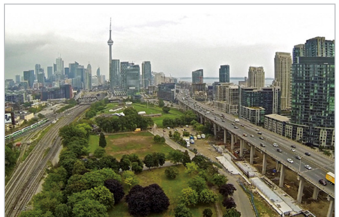
An aerial view of the fort looking east shows the substantial progress on the Visitor Centre that's been made over the summer. Photo by Danny Williams
